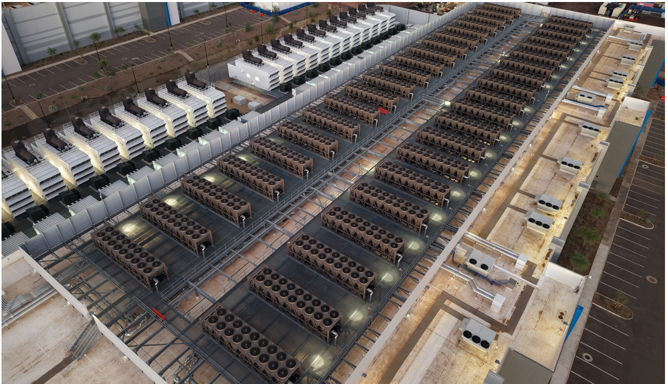
Roof of a data center showing cooling equipment and backup generators. These systems support temperature control and power continuity for high-density computing operations by managing heat and providing on-site electricity during outages. Photo by Rspark3 (Wikimedia Commons).
